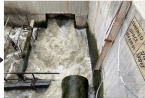
Inlet point for receiving sewage water at Eklingpura STP, Kaladwas village, Udaipur
